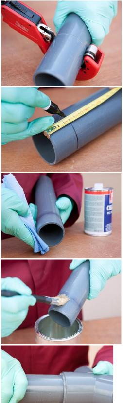
Cut the pipe end squarely, remove internal burrs and chamfer to 15°.
