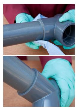
Remove the excess glue directly after the
